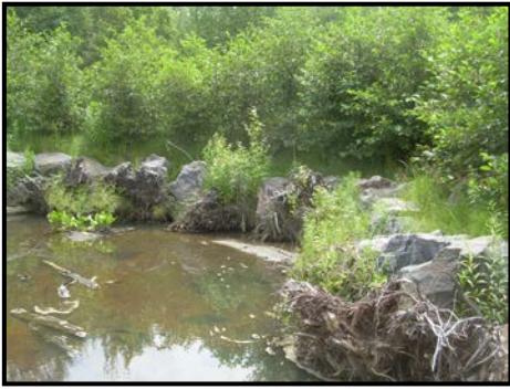
Bioengineering Root Wad Structure
