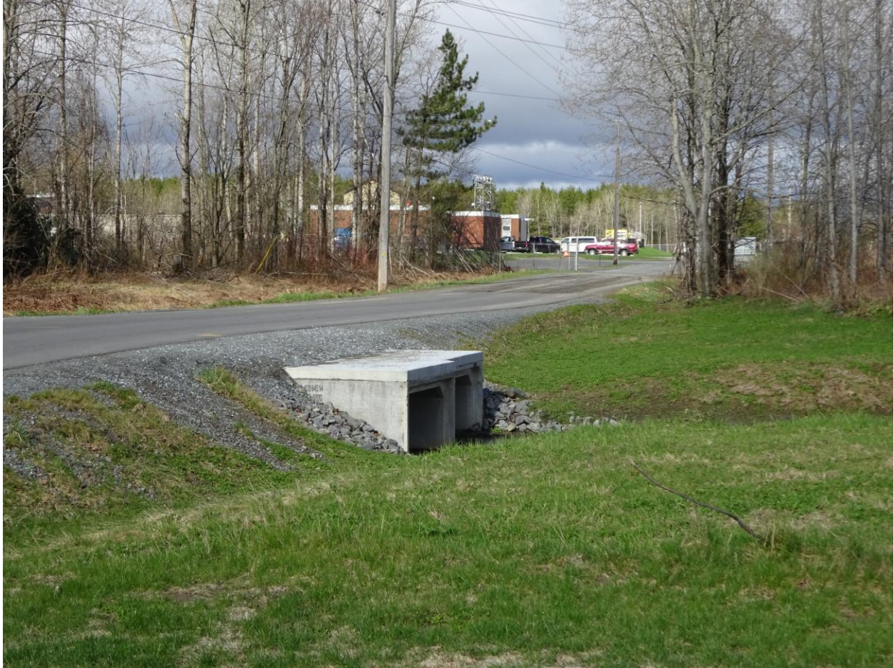
Photo 2: 1830 Yorkshire Drive, Val Caron New culvert providing drainage southerly under Yorkshire Drive File 751-7/19-1 Photography May 17, 2019
