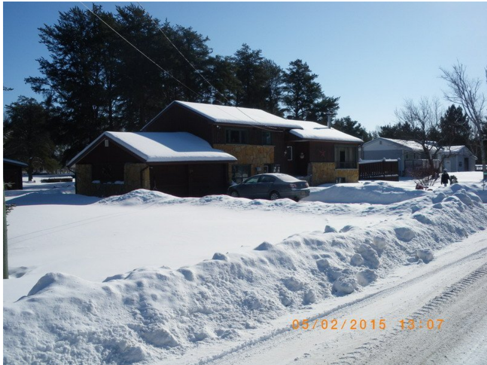
PHOTO 4 EXISTING RESIDENTIAL DWELLING TO THE SOUTH OF THE SUBJECT LANDS
