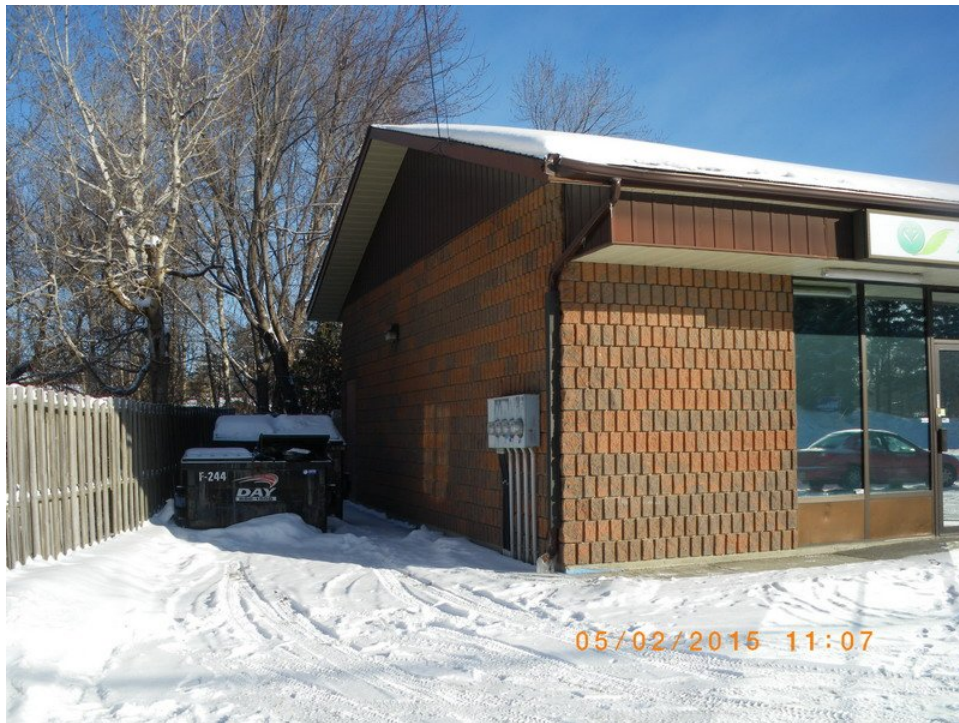
PHOTO 4 EXISTING GARBAGE DISPOSAL AREA TO THE WEST OF THE BUILDING
