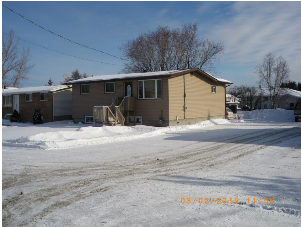
PHOTO 1 3212 HIGHWAY 69 NORTH, VAL CARON – VIEW OF SUBJECT PROPERTY FROM SIDEWALK
