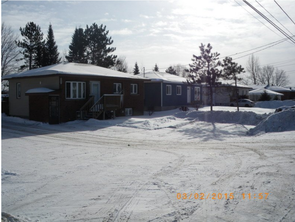
PHOTO 3 3204 HIGHWAY 69 NORTH, VAL CARON – DUPLEX DWELLING ABUTTING SOUTH
