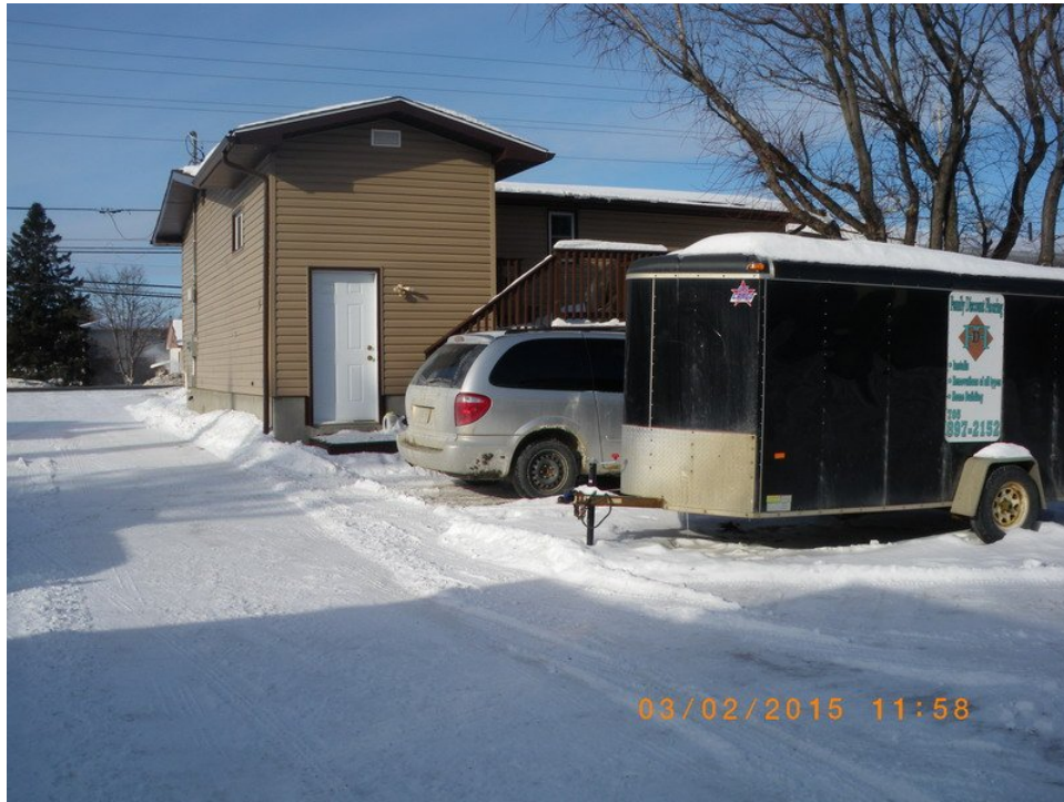
PHOTO 5 3212 HIGHWAY 69 NORTH, VAL CARON – VIEW OF REAR YARD AND REAR ENTRANCE INTO DWELLING
